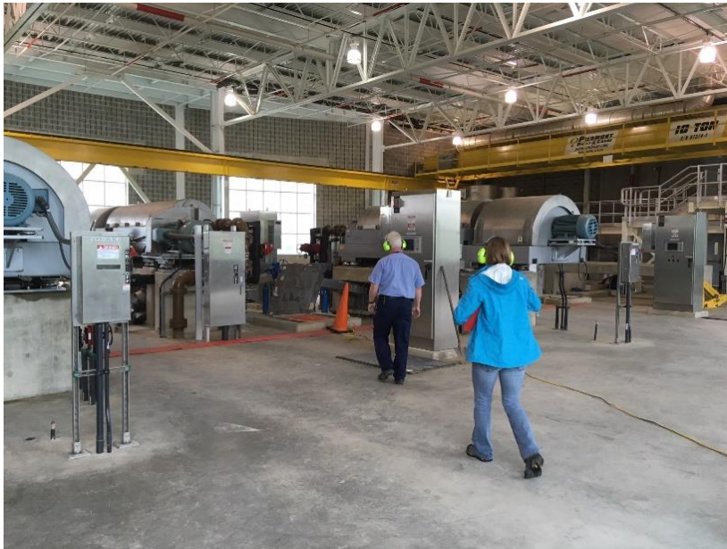
Figure WTR-1. Centrifuges used to dry WTRs at a water treatment plant
