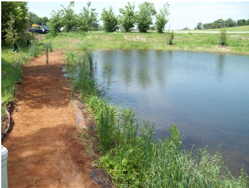
Figure IESF-7: Typical Pond-Perimeter Iron Enhanced Sand Filter
