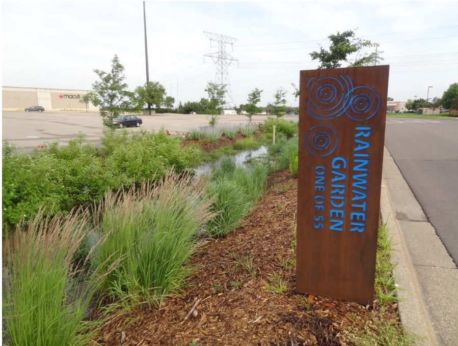
Figure IESF-8: Typical Bioretention with Iron Enhanced Sand Filter (Photo ©Barr Engineering)
