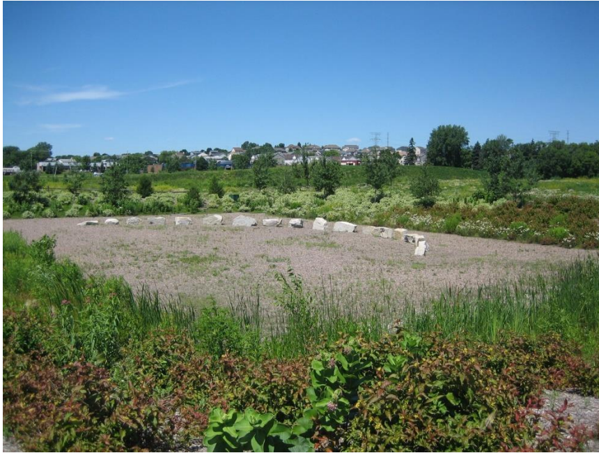
Figure IESF-6: Typical Surface Iron Enhanced Sand Filter
